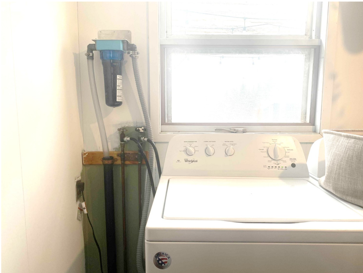
Figure 11. Example of a Lint LUV-R filter installed to a household washing machine.
