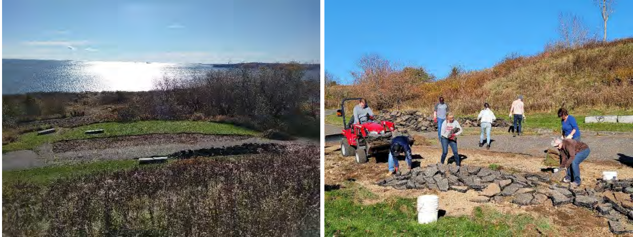
Figure 5: Volunteers removing asphalt (Left) and after completion (Right).
