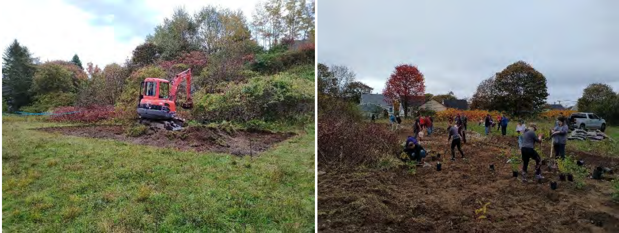
Figure 2: Montgomery Crescent rain garden construction.
