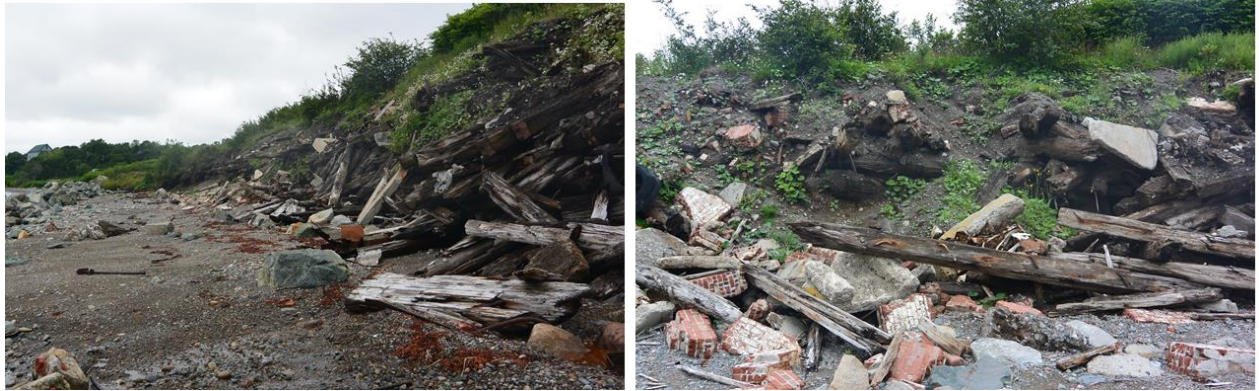
Figure 36: Image left, MCB6 looking southwest where debris is covering the slope. Right, debris in MCB6 could be from old infrastructure or infill used to extend and protect the coastline. Riprap observed along the shoreline leaving a gap between the water and debris.
