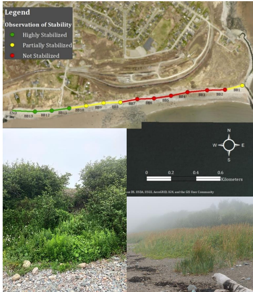
Figure 28: Observation of stability at Bayshore Beach in summer 2021. Images: left, vegetated slopes observed from BB12-END creating natural protection for residential infrastructure. Right, vegetation around public beach access in BB11 before slope increases where residential development is observed.
