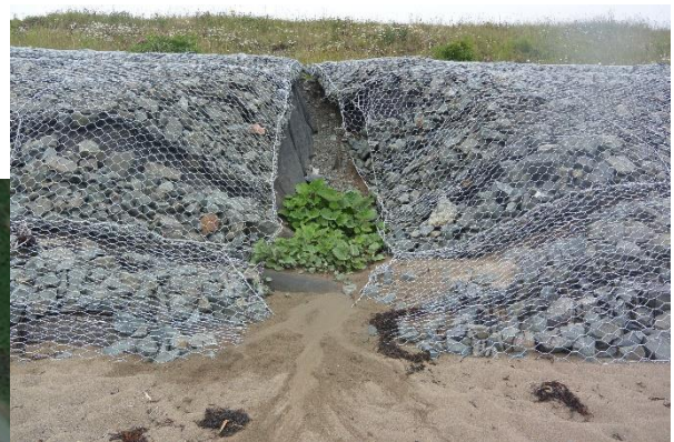
Figure 11: Left, form types along Mispéc Beach observed summer 2021. Image above, showing a drainage channel in the riprap where repairs may be required.
