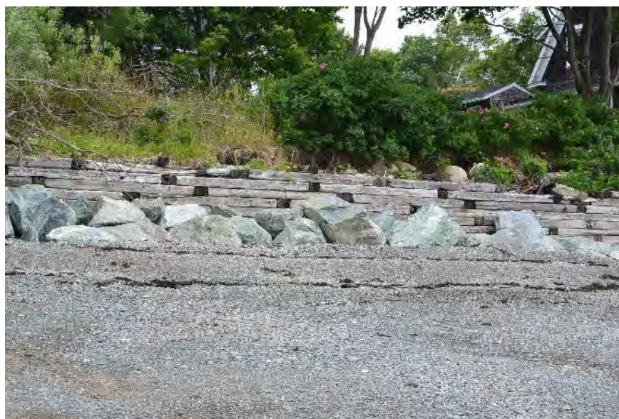
Figure 15: A series of two hard protection methods put in place by a local resident along McLaren's Beach. Closest to the shore is a small layer of stone and then behind that, a wooden seawall built to protect the coastline from wave action. Just above the wooden sea wall, the bank has been undercut by large wave events leaving bushes hanging overhead (ACAP Saint John, 2016).
